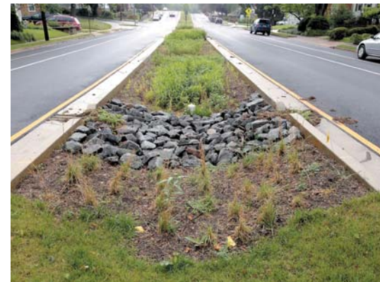
This bioretention area is the first of many to be installed across Arlington County.
