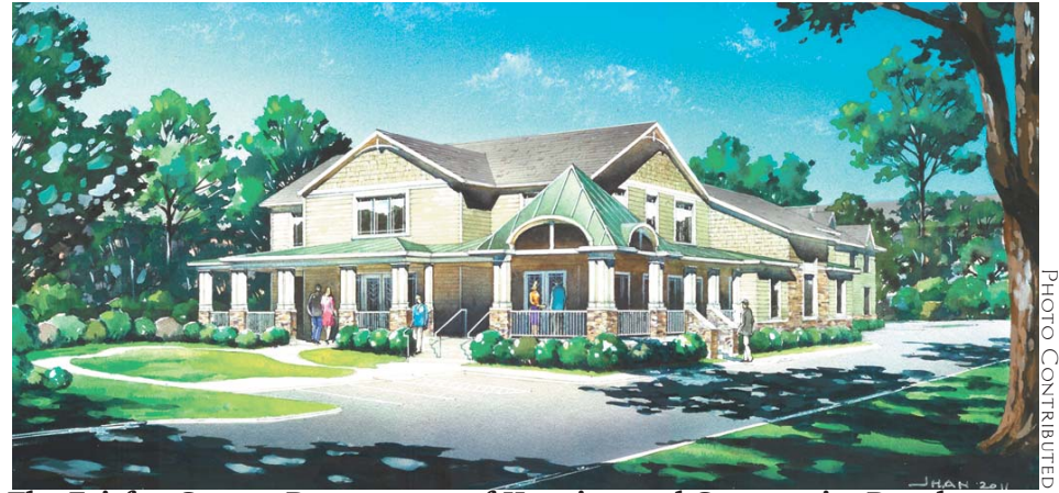
The Fairfax County Department of Housing and Community Development (HCD) is developing the "Residences at Mondloch" in partnership with the Fairfax County Office to Prevent and End Homelessness, New Hope Housing, and other community partners.
