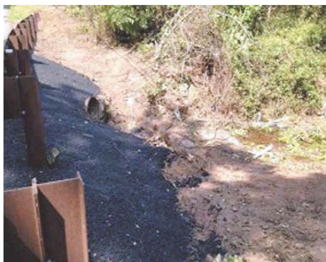
MC-DOT paving up to stream edge increasing run-off
