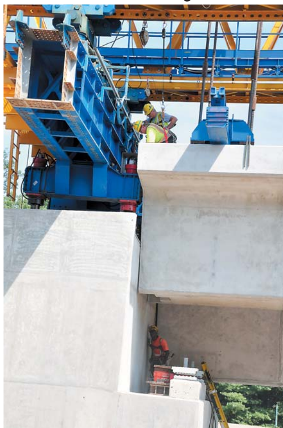
Workers lower the final aerial span for the Metrorail track in Tysons Corner Tuesday, July 17.
