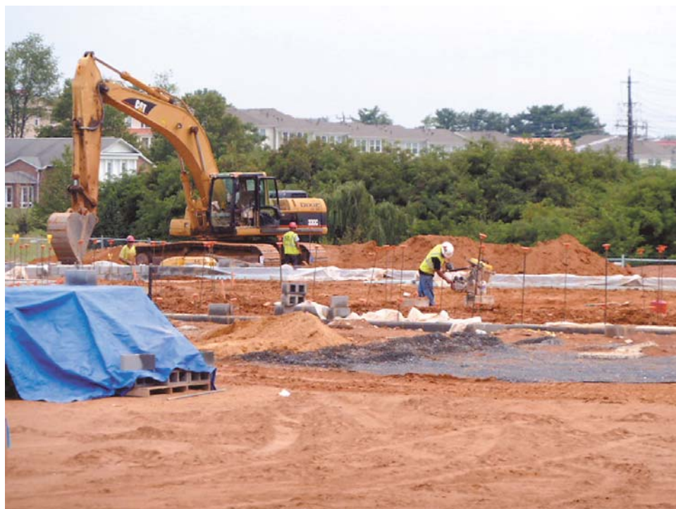
The foundation being laid at the Animal Services Center.
