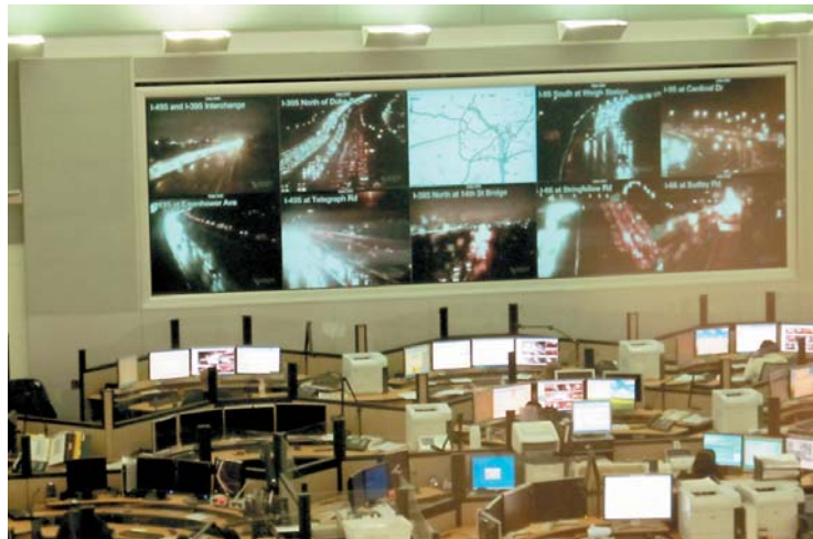
Fairfax County's 911 Call Center located in the McConnell Public Safety and Transportation Operations Center, named after former Fairfax County Supervisor Elaine McConnell.
