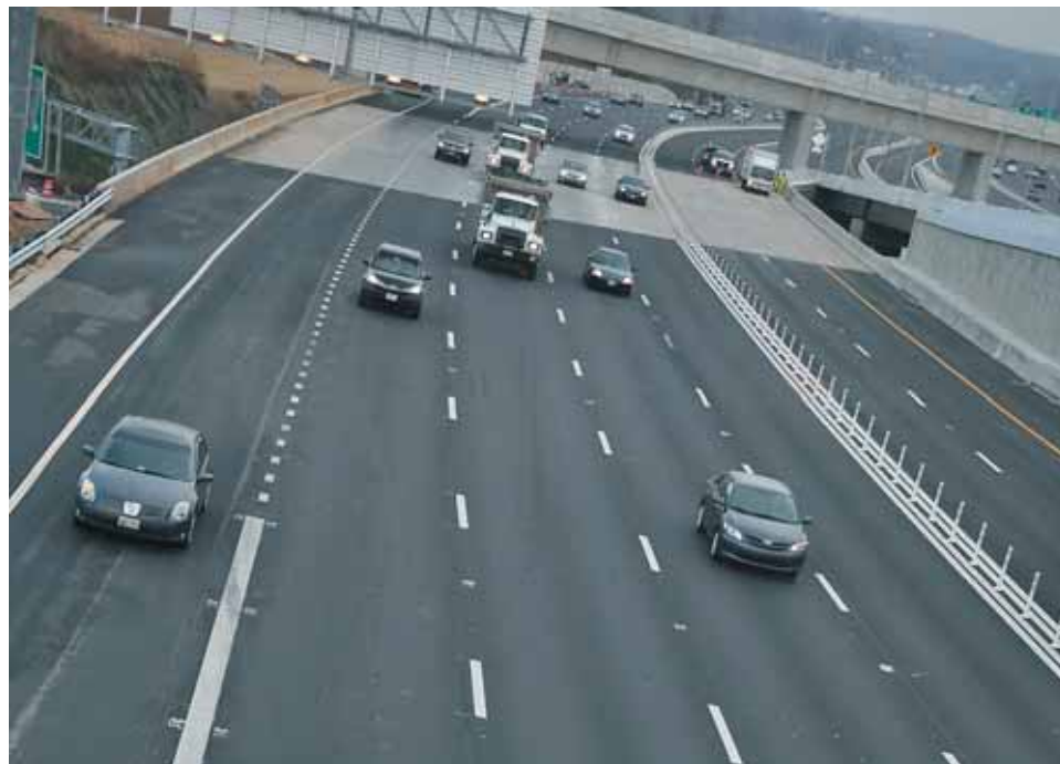
The 495 Express Lanes opened Saturday, Nov. 17, providing two new toll lanes over 14 miles of the Beltway from the Dulles Toll Road to Springfield.
