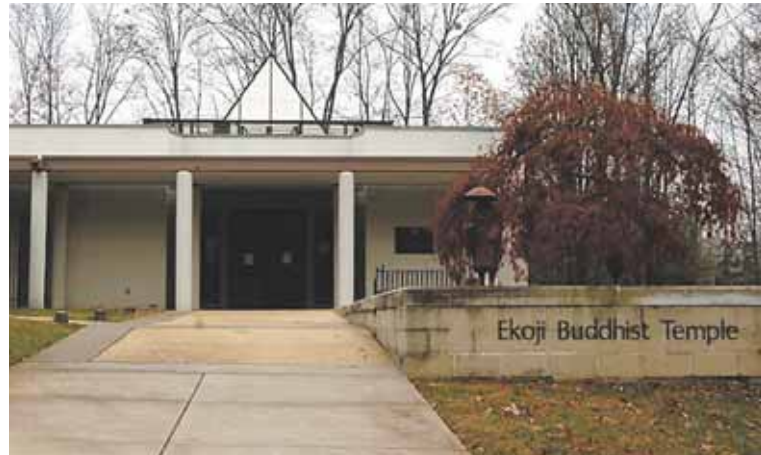
PHOTO BY MARGARET JOHNSTON/THE CONNECTION The Ekoji Buddhist Temple in Fairfax Station.
