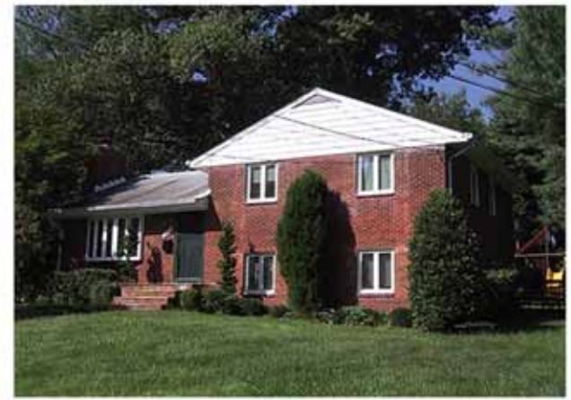
Before an Addition
