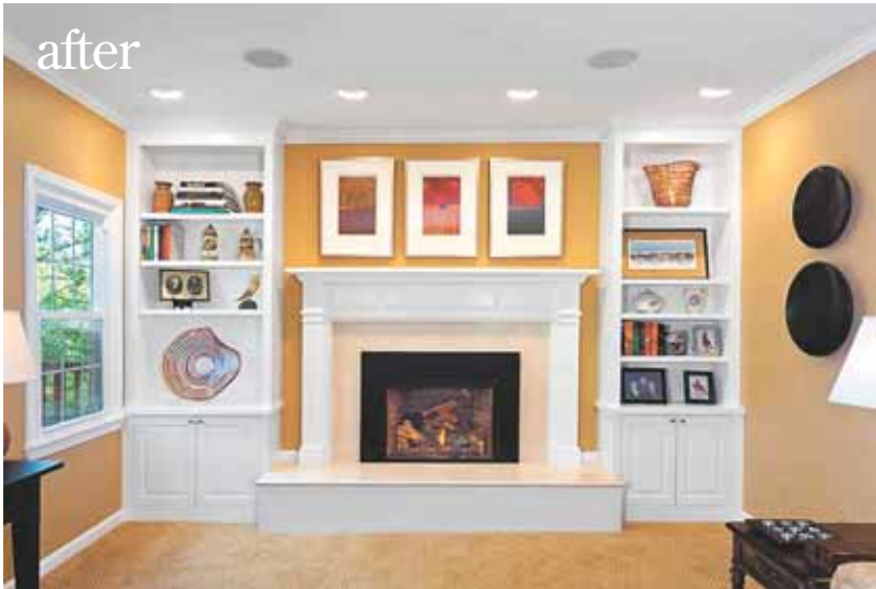
The existing half-brick floor-to-ceiling backwall was replaced by perfectly symmetrical built-ins, crown molding and an elevated hearth with a marble surround and Edwardian-style mantle.
