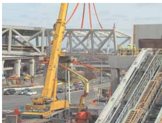
Crews complete the installation of the last segment of the pedestrian bridge that connects the Tysons Corner Station with the pedestrian pavilion near Tysons Corner Center. Framework for pavilion escalators is pictured on the right.
