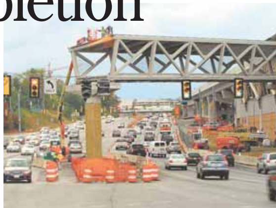
Preparing for the installation of the second segment of pedestrian bridge at McLean Station along Route 123.
