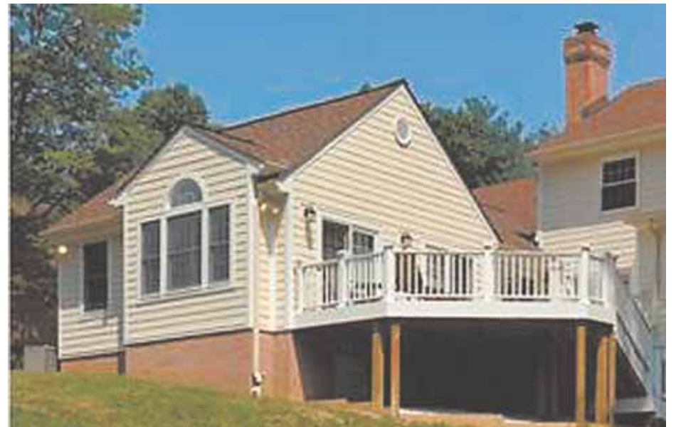
The addition of a main-level master suite with easy access to outdoor living space paves the way for aging in place and family entertaining.
