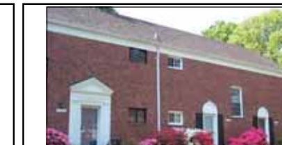
Alexandria 3456 Martha Custis Drive #312 $249,900 Freshly painted, bright and sunny, end unit. 605 sq ft top unit with replaced vinyl windows, newer heaters and ac's. Updated kitchen. Washer/dryer. Refinished parquet flooring. Upgraded electrical panel. Attic storage. Rita Tassa 703-629-8624
