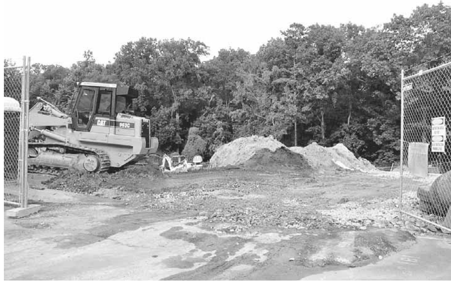
The Scotland Community Center is under construction and set to open next summer.
