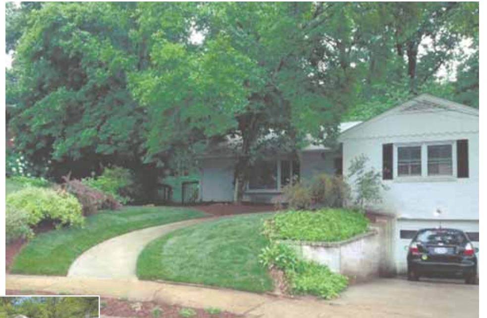
When Jaime Marquez began having difficulties getting from the house to the driveway, Glickman Design Build created a graduated front walk for the Arlington family. The new walk rises one inch per foot. The plan included replacing a front stoop with a "zero step" entry and widening interior doors and halls.
