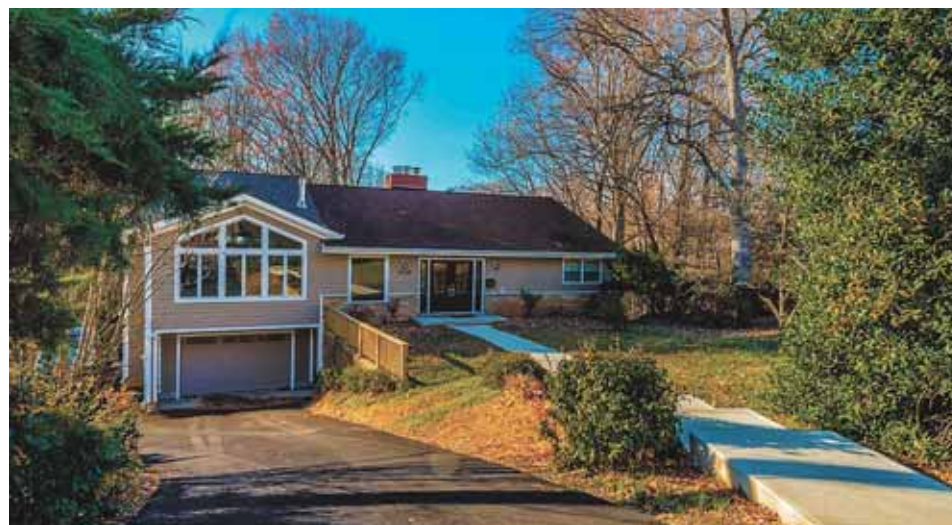
The 17.5-foot by 13-foot window wall that dominates the new side-facing gable is one component in a renovated front elevation which now features a well-defined entranceway comprised of glass-facing French doors and sidelights.
