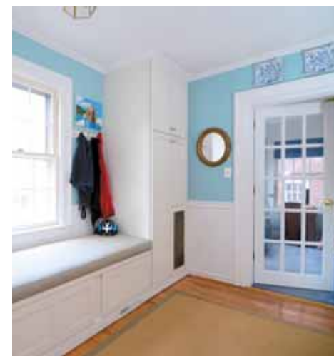
The renovation of this Arlington, Va., home includes a new mudroom with window seat storage and a door to the separate office space.
