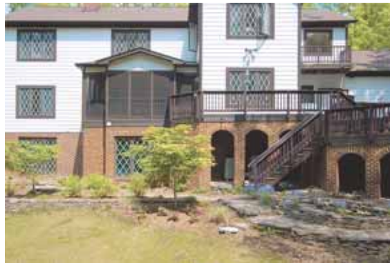
PHOTO COURTESY OF FOSTER REMODELING SOLUTIONS
