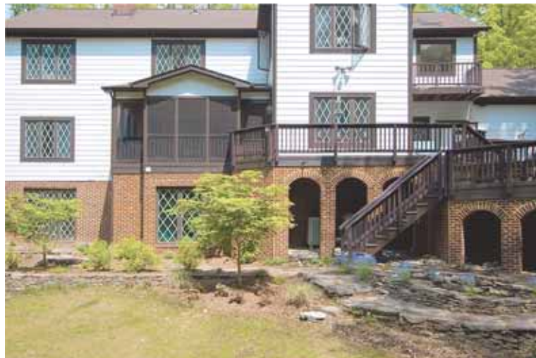
PHOTO COURTESY OF FOSTER REMODELING SOLUTIONS
