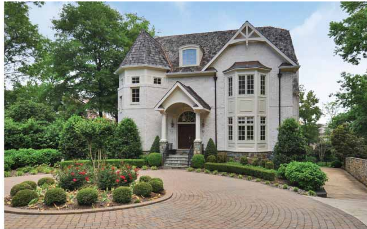
WELLINGTON $2,950,000 | ttrsir.com/id/FX8249143 This French Country Chateau features stunning views of the Potomac River. 8,500 square feet of elegant living space on .61 acres of beautifully landscaped grounds. Six large bedrooms and four+ baths on four levels. PHYLLIS PATTERSON +1 703 408 4232 BRITT PATTERSON +1 703 517 0630
