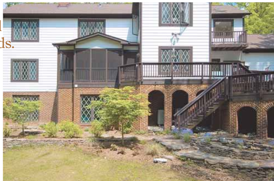
PHOTO COURTESY OF FOSTER REMODELING SOLUTIONS
