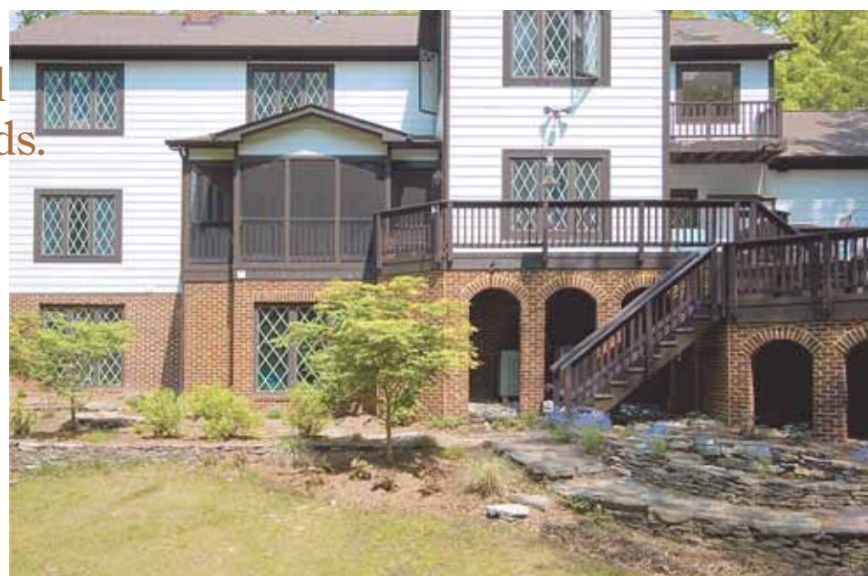
PHOTO COURTESY OF FOSTER REMODELING SOLUTIONS
