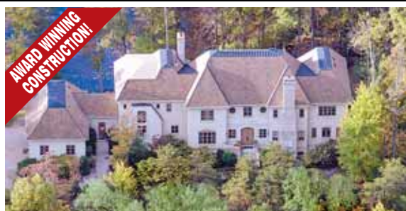
AWARD WINNING CONSTRUCTION! Great Falls $3,148,880
