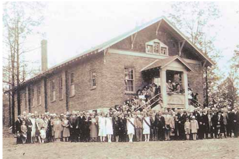
The Great Falls Grange Hall, opening day: May 4, 1929.
