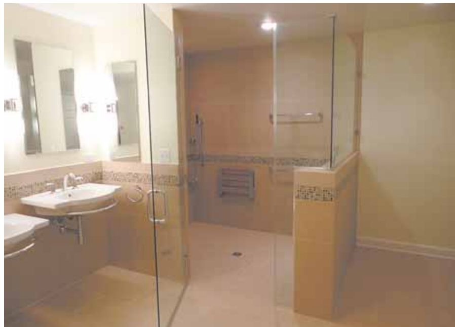
The curbless roll-in shower was designed for wheel-chair access.
