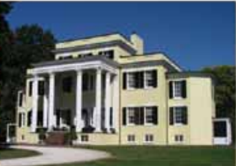
Historic House & Gardens
