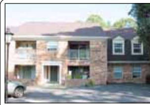
Burke Cove Condo $1,450 Beautiful Burke Centre Beautiful New Renovation/Upd ates to include Kitchen & Bathroom - New
