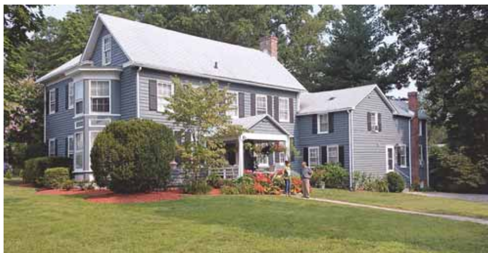
The front of the Ashland House. Standing in front are guides, Jumana Qamruddin and Nazir Bhagat. Bhagat, who owns the house, purchased it in the 1980s and has done extensive research on the history of the house. The house is complicated in structure, featuring several add-ons. Guests reported that going through the house felt like walking through a maze. The front and back stairs of the house are reminiscent of Greek Revival Style, according to Bhagat.
