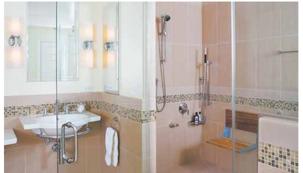
When remodeling this bathroom, Glickman Design Build added a bench to this shower. Such features can help seniors to downsize and live alone safely.
