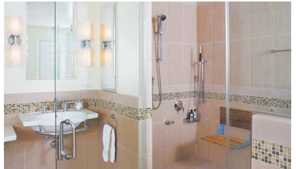
When remodeling this bathroom, Glickman Design Build added a bench to this shower. Such features can help seniors to downsize and live alone safely.
