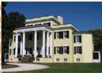
Historic House & Gardens
