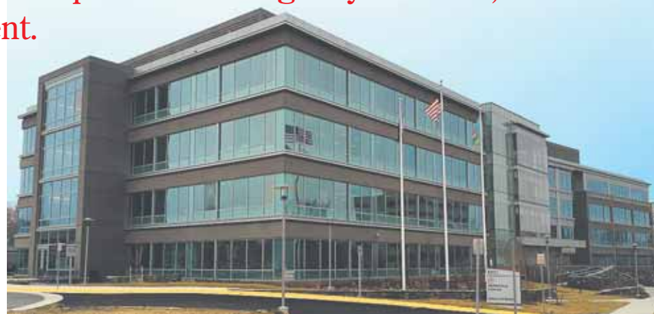
Fairfax County Community Services' Board opened its new facility in Merrifield.
