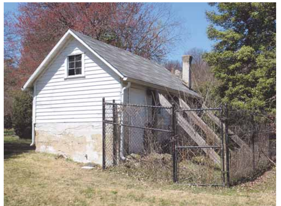
Milk shed on the Reeves property with wooden structural supports installed by Arlington County.
