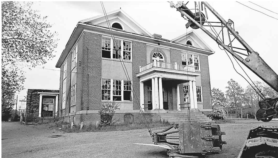
Original building being razed.
