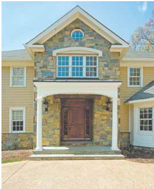
The new portico lends needed definition to the entrance way of the Jeff and Sharon Roman’s Great Falls home. The metal-clad roof is visually unified with a garage overhang supported by decorative brackets.
