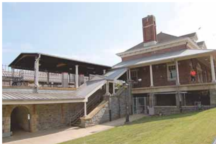
The tunnel and the station on King Street.
