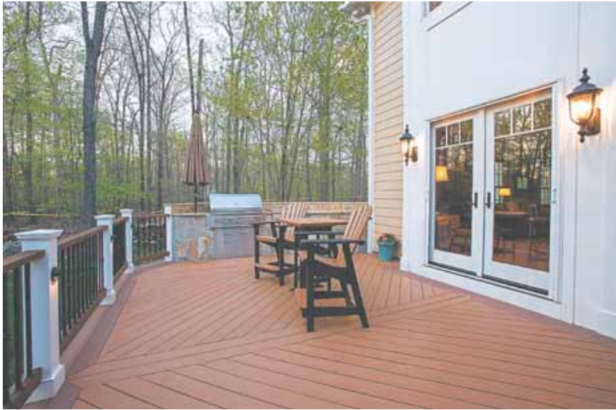
To assure the durability of the deck's surface, Sun Design specified Trex planking instead of wood, and narrowed the span between joists from 16 inches to 12 inches.
