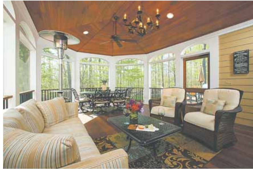
The spacious new screened porch demonstrates how highly durable materials can be shaped to meet demanding aesthetics. The Ipe decking chosen for the porch flooring is one of the one of the most enduring natural hardwoods offered for outdoor surfaces; installed in a tongue-and-groove pattern, it keeps out bugs more effectively than screen mesh. The fiberglass charcoal screen, likewise, makes it hard to see the porch interior from the outside.
