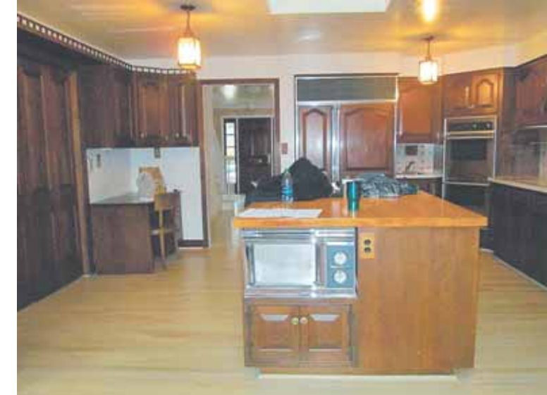
BEFORE: The existing kitchen's dated Colonial accents included Dutch-style maple cabinet facings, a mosaic tile back splash and a vinyl counter surface.
