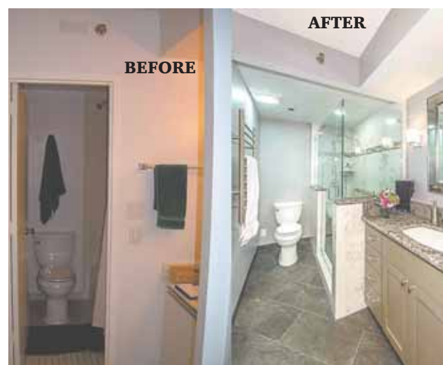
Recognizing that inches count in a tight footprint that can't be expanded, Sarah Wolf at Foster Remodeling Solutions gained just two inches of floor space by removing a wall between the vanity and the tub (left); the half-wall and frameless glass space divider that now surrounds the newly installed walk-in shower (right) invites line of sight that previously didn't exist.
