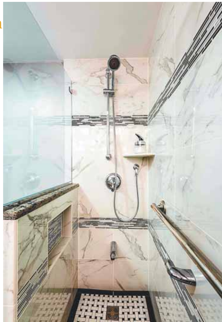
The black and white art deco-style ceramic basket-weave pattern for the shower prevents slipping. As an aging-in-place consideration, Wolf, of Foster Remodeling, found room for an in-shower bench and grab bars. A hand-held shower head on a slide bar adjusts to the owners' different height requirements.
