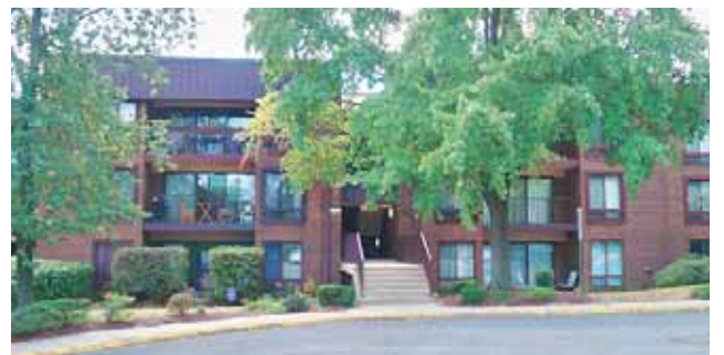
Fort Ellsworth 134 Roberts Lane # 403, Alexandria VA Top floor unit in immaculate condition! Brand new neutral carpet & ceramic tile floor in kitchen. Neutral paint color. New custom windows & balcony door. W/D in unit. Pkg space. $258,000 Wendy Smith MLS # AX8743185
