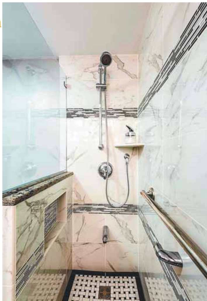
The black and white art deco-style ceramic basket-weave pattern for the shower prevents slipping. As an aging-in-place consideration, Wolf, of Foster Remodeling, found room for an in-shower bench and grab bars. A hand-held shower head on a slide bar adjusts to the owners' different height requirements.
