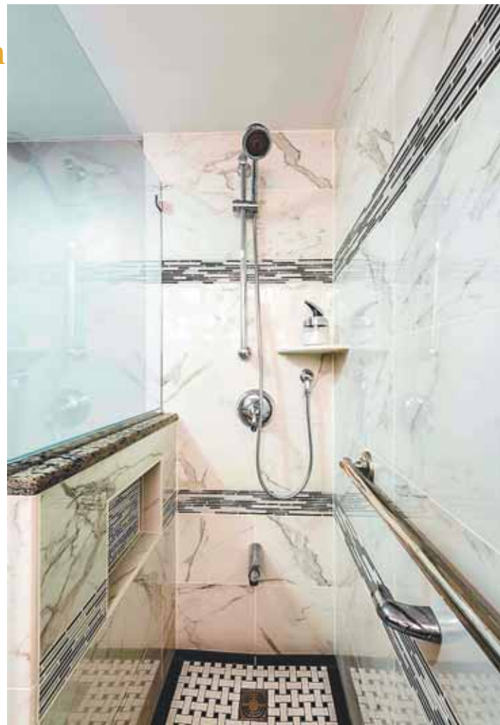
The black and white art deco-style ceramic basket-weave pattern for the shower prevents slipping. As an aging-in-place consideration, Wolf, of Foster Remodeling, found room for an in-shower bench and grab bars. A hand-held shower head on a slide bar adjusts to the owners' different height requirements.
