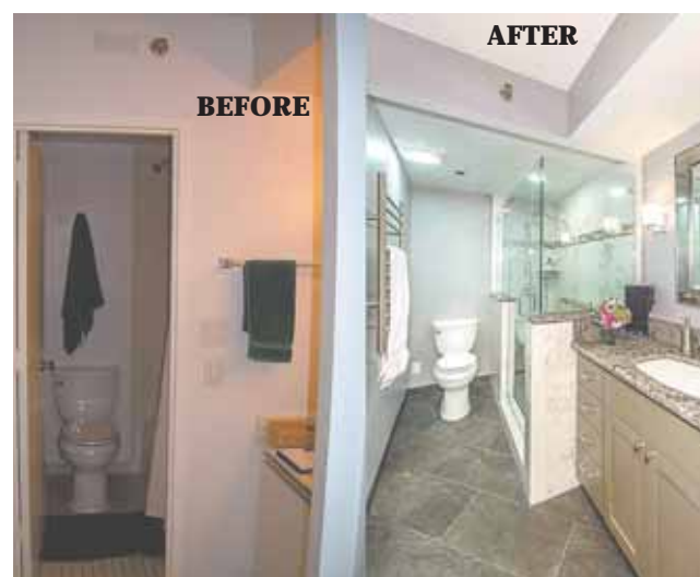
Recognizing that inches count in a tight footprint that can't be expanded, Sarah Wolf at Foster Remodeling Solutions gained just two inches of floor space by removing a wall between the vanity and the tub (left); the half-wall and frameless glass space divider that now surrounds the newly installed walk-in shower (right) invites line of sight that previously didn't exist.
