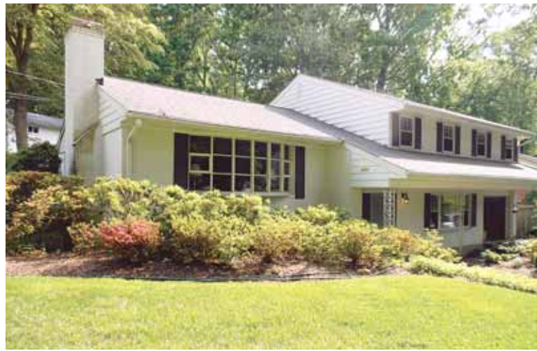
Before: The roof overhang to this circa-1960's split-level was thought to restrict any practical consideration to redesigning the home's front elevation. On two occasions, the family hired architects to develop a solution, but nothing feasible resulted.
