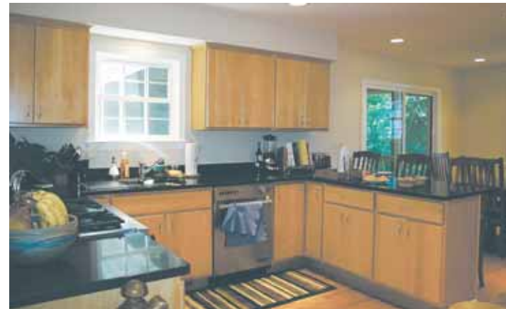
The first phase of a 10 year remodeling plans entailed replacing the kitchen/living room divider wall with a dining counter/serving station. The revisions allowed light from three directions. Maple cabinets and Silestone quartz surfaces provide a tonal and textural contrast.
