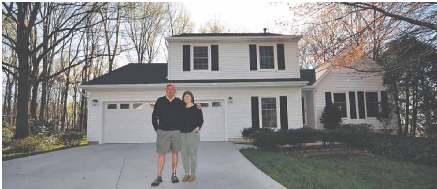
Mike and Sandy Nusbaum have enlarged their home four times in the past ten years. Each phase has improved the home's overall functionality, which has transformed it into a preferred gathering place for children, grandchildren and extended family. The garage and storage units have resulted in a dramatic improvement in available space and eliminated clutter.
