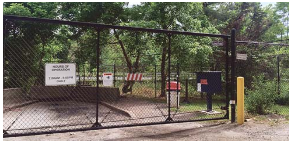
The Colvin Run Septic Sewage Receiving Plant site will close on June 27 due to safety and access issues related to the Difficult Run pump station project, according to Matthew Kaiser, with Department of Public Works. Rehabilitating the site would not address the issues of safety on the road/trail, flooding, and the lack of queuing space and a turn-around lane, according to county documents.
