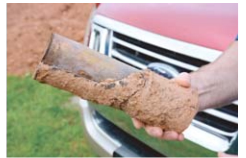
Kabat holds a segment of copper pipe inside iron that was found beneath an old white oak tree on the Silas Burke House property. It may have been an old iron sewage pipe that went to a septic tank.
