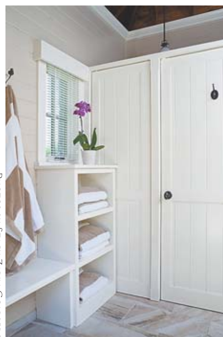
To keep down moisture build-up, the tongue-and-groove interior walls were milled in a specialty woodworking shop, spray-painted and treated under shop conditions, installed on-site, then painted again in a bright white enamel formulated for kitchen cabinets. The light gray porcelain tile conceals radiant flooring.
