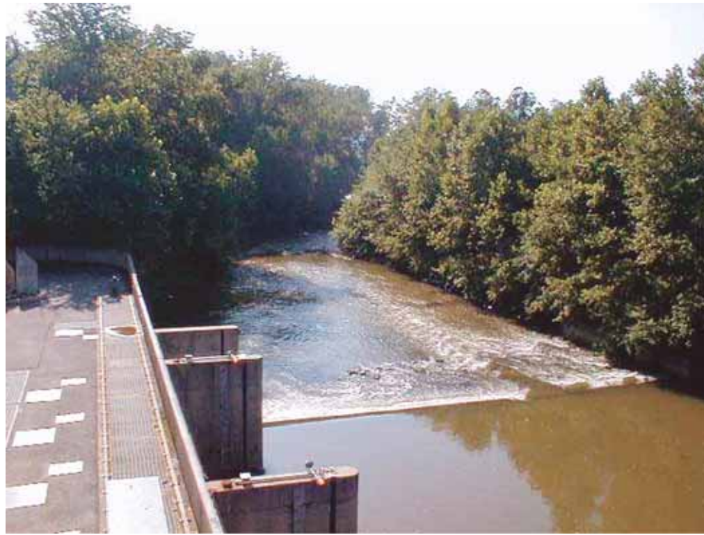
The Potomac Filtration Plant's current intake.
