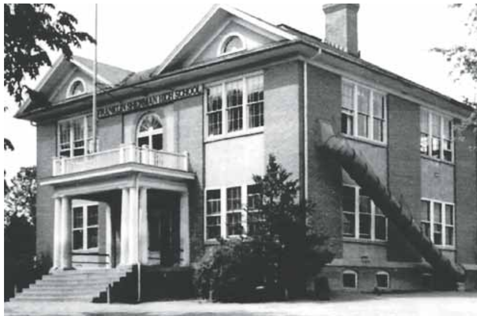
The Franklin Sherman School opened in 1914 facing what now is called Corner Lane.
