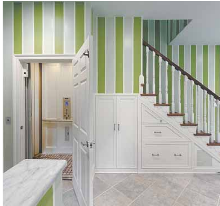
An existing closet space or other small area can be retrofitted to accommodate an elevator.
