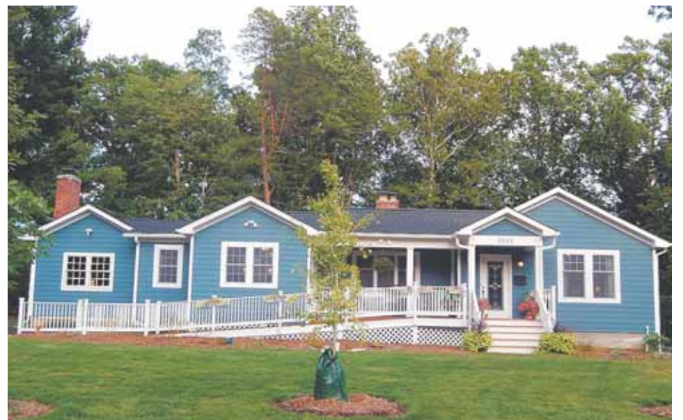
There's a long ramp in front of the home on Burrows Avenue.
